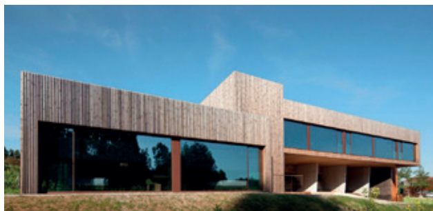
照片: José Campos Architectural Photographer
